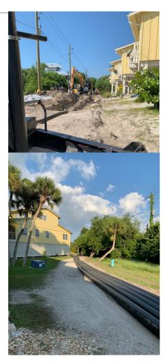
suppression system in 'A' bldg. The water main has been repaired & the fire system has been tested by an authorized contractor to ensure the system is fully operational.
